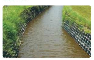
Corys Geosynthetics geocell products are three- dimensional, expandable panels made from high-density polyethylene (HDPE), polyester or other polymer materials.
