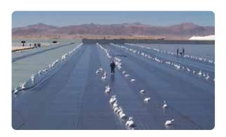
Corys Geosynthetics branded HDPE, LLDPE, FPP, TPO and VLDPE liners.0.75 mm to 3.00mm thickness in both smooth and textured form.
