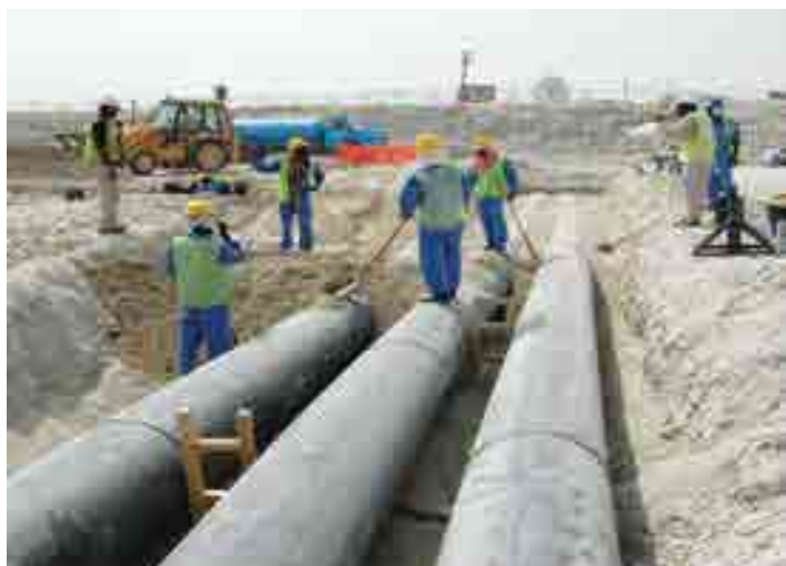
Figure 2-Typical Open Trench
